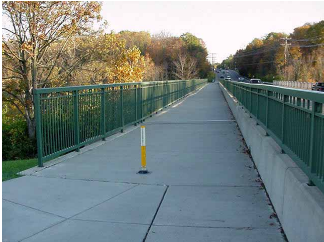
Figure 25: Railings on a Shared Use Path
